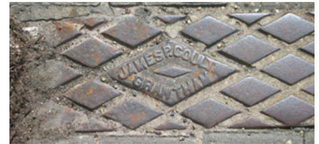
Figure 8.1.41; Locally produced manhole covers
