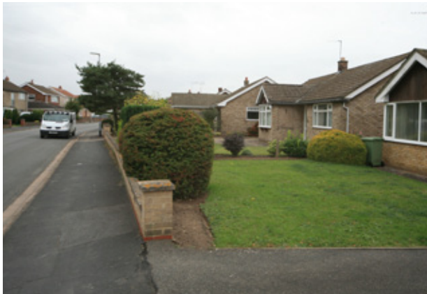
Figure 8.6.07; Single storey dwellings are usually grouped to particular roads (CA06c)
