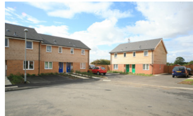
Figure 8.10.11 and Figure 8.10.12; Older and relatively recent housing within CA10 follow a simple vernacular. Note the use of weatherboarding to the new houses (not a local tradition)
