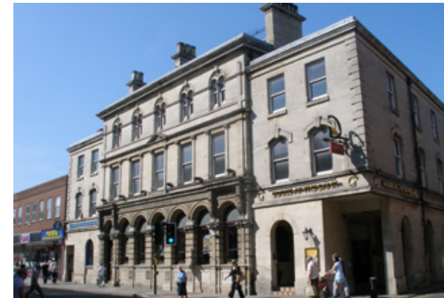
Figure 8.1.22; Former banking halls, High Street (CA01b)
