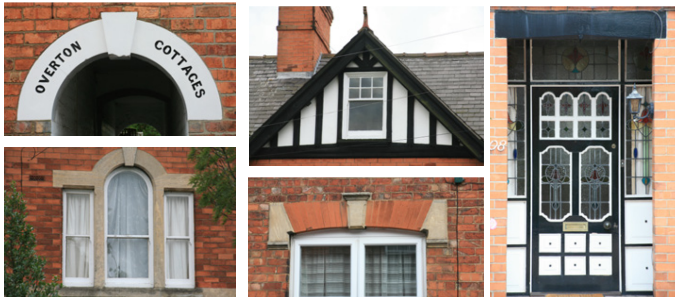
Figure 8.10.16; An eclectic mix of Victorian and Edwardian detailing can be found to some parts of the character area, most notably CA10d
