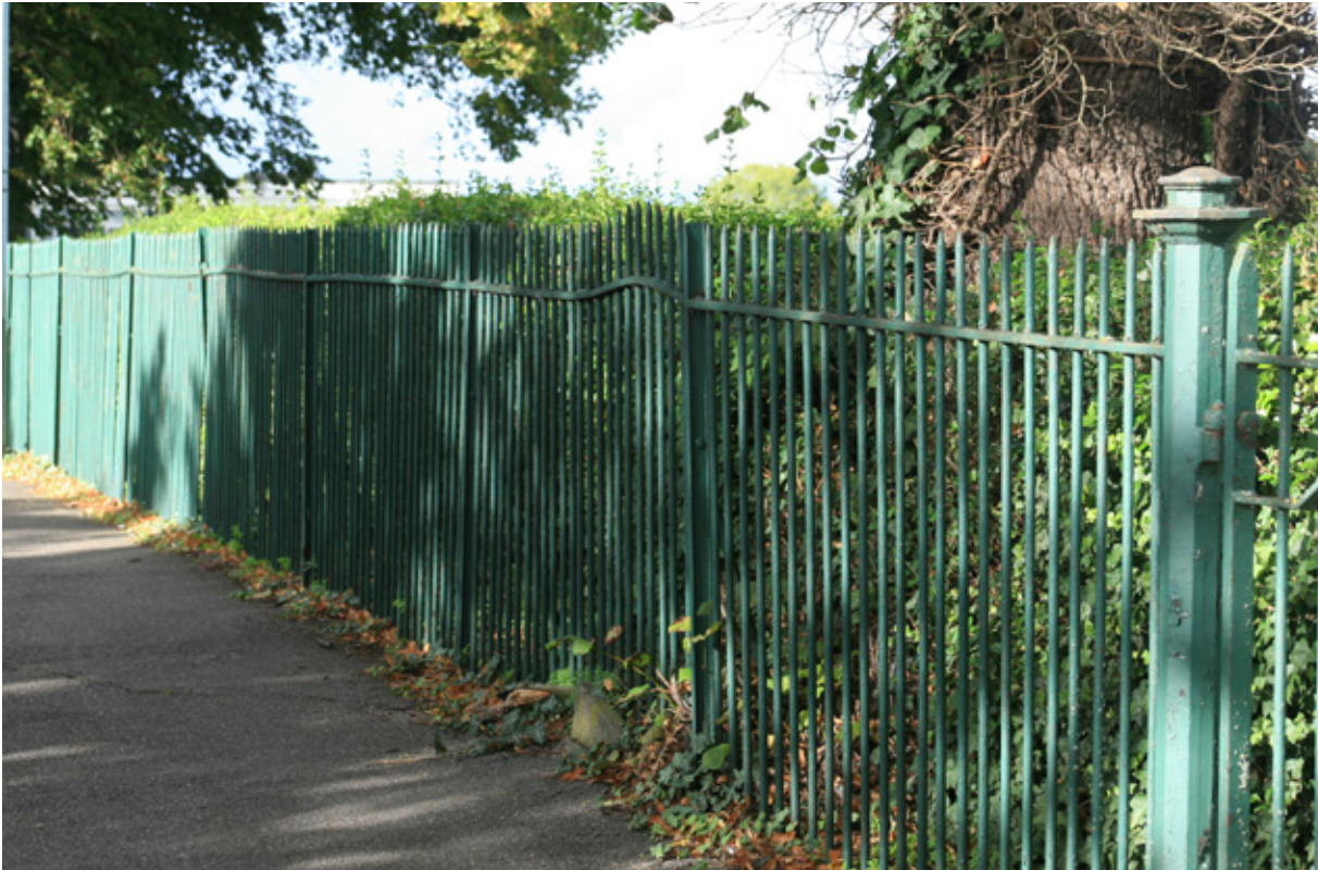
Figure 8.4.16; Cast iron railings define the pavement edges to parts of Stonebridge Road
