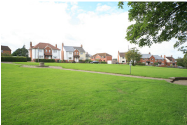
Figure 8.7.08 and Figure 8.7.09; Housing in the spirit of the Garden city movement with generous green open space (off Harrowby Lane – CA07b)
