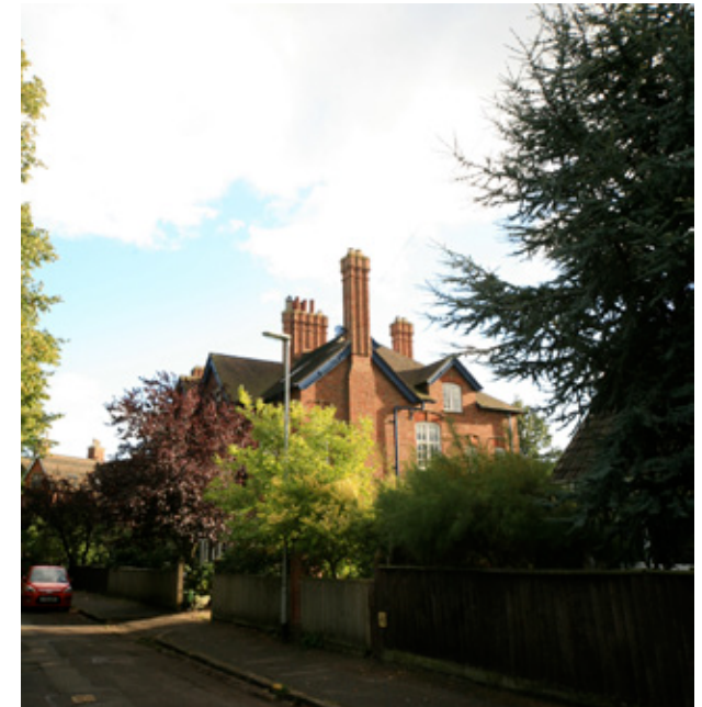
Figure 8.2.17; Trees play an important role of framing and sometimes obscuring houses from view in Welby Gardens (CA02c)
