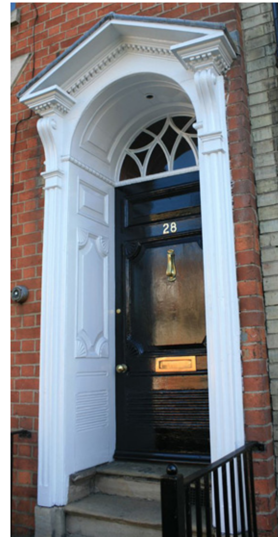
Figure 8.2.13; Decorative joinery, particularly doorcases, is a common feature to houses in CA02a (North Parade)
