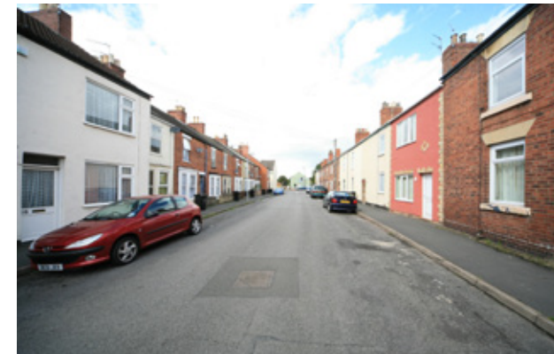
Figure 8.3.15; Some red brick houses have been rendered and painted and some have lost original windows destroying the unity of the terrace
