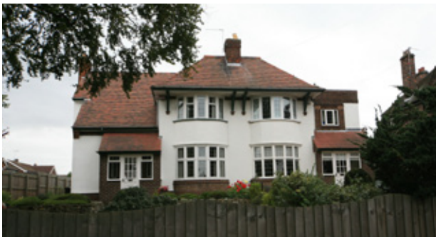
Figure 8.6.14; Brick, render and clay tile are characteristic of Manthorpe Road
