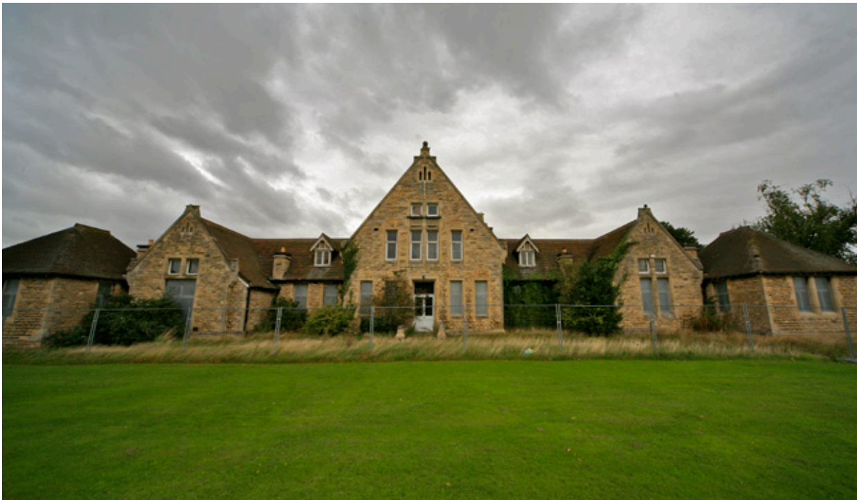
Figure 8.6.13; The Victorian range of buildings comprising the original Grantham Hospital (presently boarded and in a poor condition). These buildings are considered important heritage assets worthy of retention and re-use.
