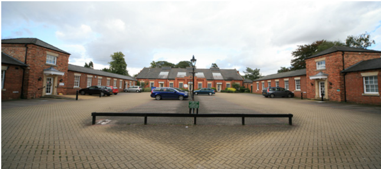
Figure 8.4.08; Former Grade II listed military barracks now converted to business units
