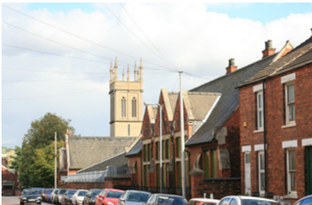
Figure 8.3.31 and Figure 8.3.32; Views to St John's Tower, Station Road
