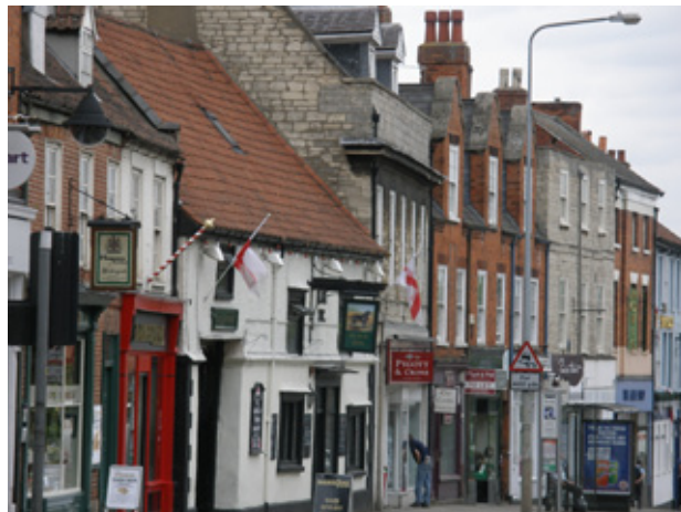
Figure 9.01; The rich variation to the townscape of Watergate exemplifies the quality of the built form in Grantham
