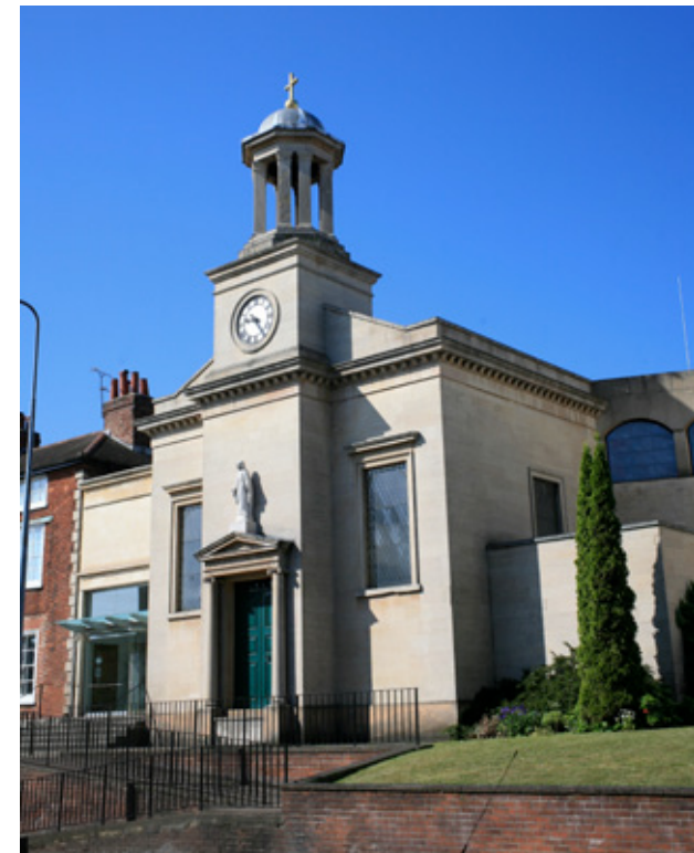
Figure 8.2.14; The church of St Mary – an exception to the red brick of the adjacent terraces. Its modern extension is sympathetic and well-handled architecturally.
