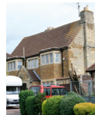
Figure 8.7.15; Older farmhouses and some early houses have been subsumed by later development. There is a good use of locally distinctive materials to these earlier buildings.
