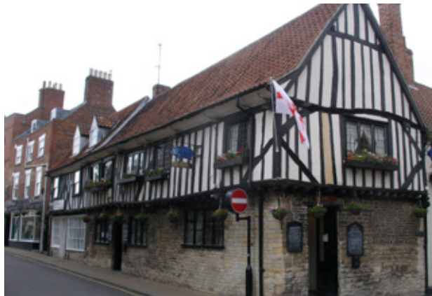
Figure 8.1.25; Public houses – timber-framed
