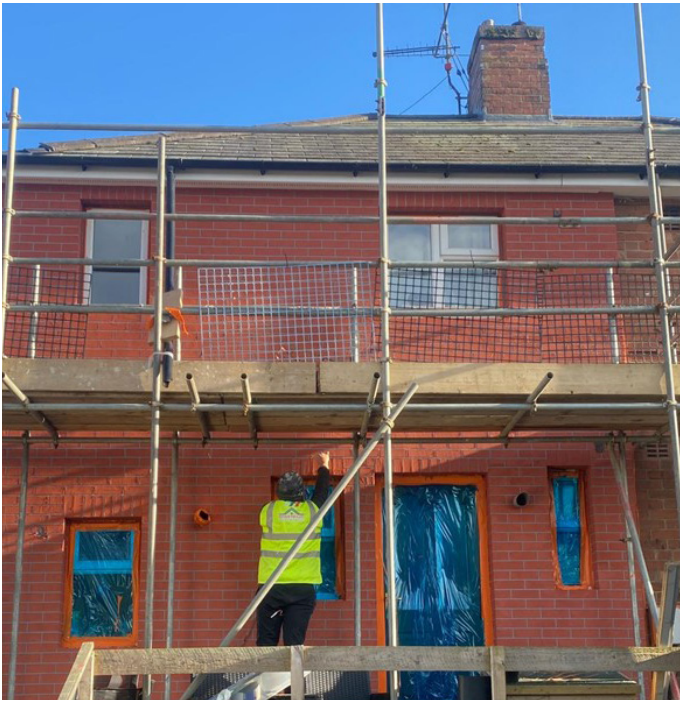
External wall insulation being installed at properties across South Kesteven
