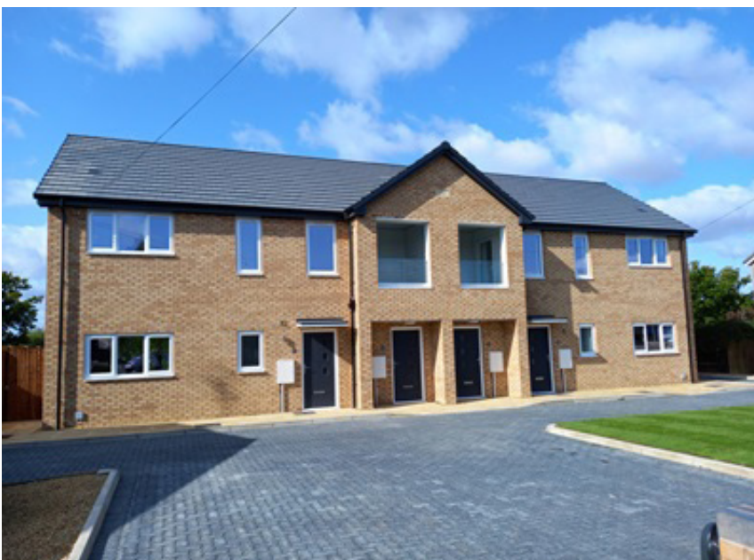
The finished homes at Elizabeth Road, Stamford.
