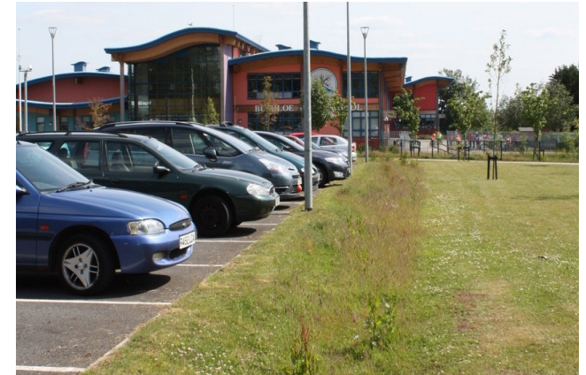
Figure 17: Shallow car park swale with very high infiltration in Bushloe High School in Wigston, Leicestershire (Image credit: DSA Environment + Design)
