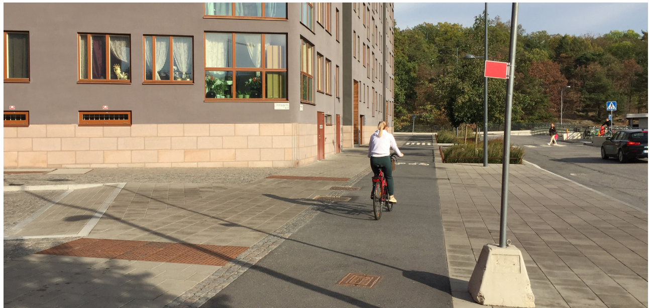
Figure 38: Raised cycle and pedestrian paths at entrance to new development making it clear who has priority.
