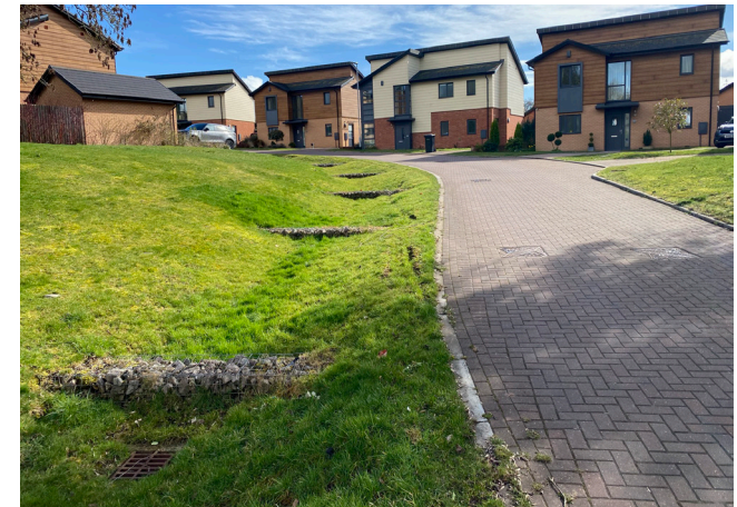
Figure 18: Award-winning roadside swale in Lincoln
