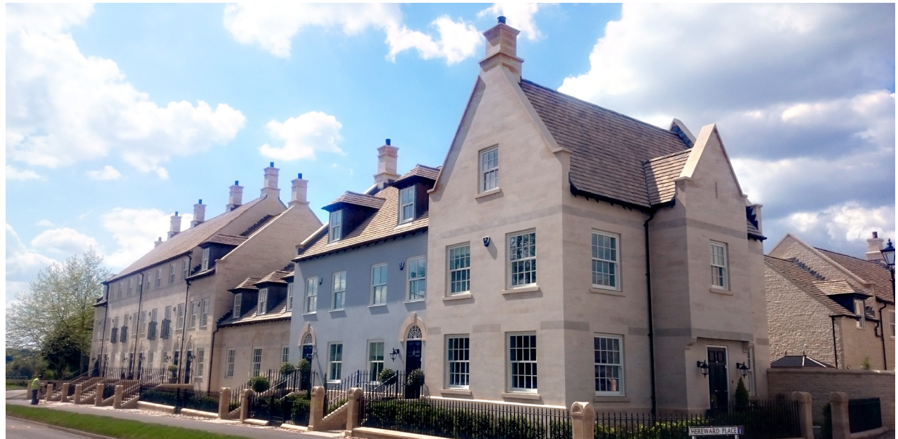
Figure 44: Cecil Square, Stamford. Variations on a pitched roof theme offering variety and unity at the same time.
