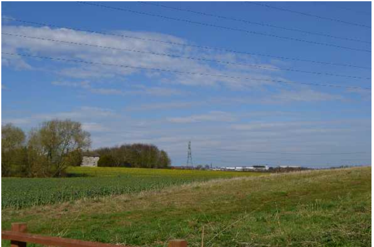
Figure 40: Area 4 land south of listed Harlaxton Lower Lodge (pictured), forming part of its setting and visible from it, therefore not suitable for development. However, note extensive planting to east of lodge screening its views of Grantham and the A1
