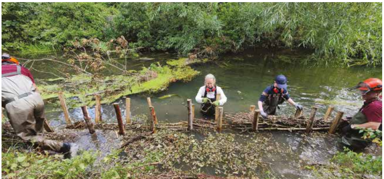
Volunteers working on a new berm in Queen Elizabeth Park
