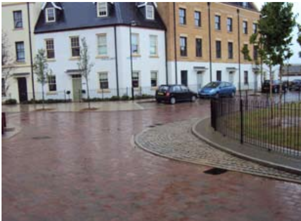
Upton, Northampton has also delivered high quality public realm improvements and new open spaces as part of the medium density housing offer
