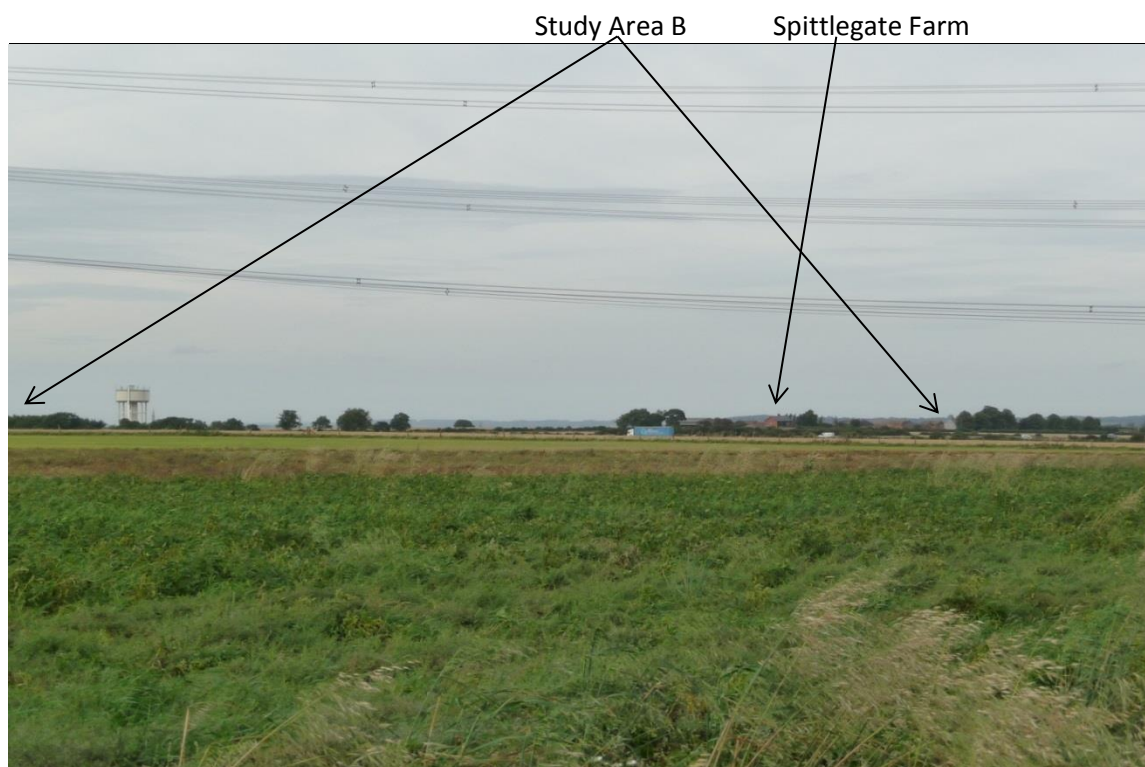
Photograph 10: from a public footpath to the south, showing the southern edge of Area B beyond the A1. The water tower, Spittlegate Farm and isolated properties lie close to the ridge of high ground along Gorse Lane which screens views of the town.
